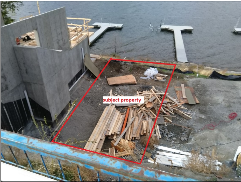
Figure 4: East View of Subject Property (from Lakeside Road)
